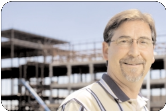
Clint Holdsworth in front of construction for the expanded production facility at the Vacaville plant. The water system at this facility is being designed with conservation in mind and is expected to save 20 million gallons per year.
